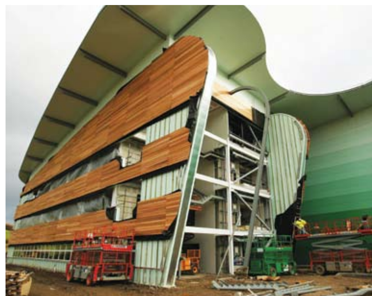
Finishing work under progress
